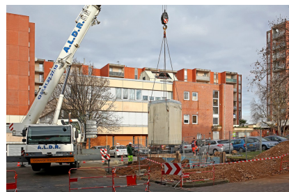
INSTALLATION DE CONTENEURS ENTERRÉS
