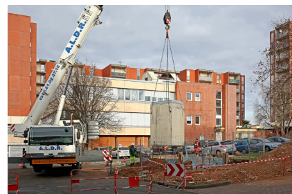
INSTALLATION DE CONTENEURS ENTERRÉS
