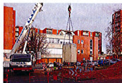
INSTALLATION DE CONTENEURS ENTERRÉS
